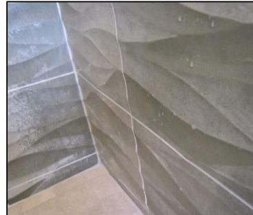
Photo # 64 Improper specification of material - very porous material in a wet area - correct: multiple sealing applications on multiple days
