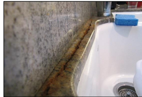
Photo # 60 Blown rod from using metal in wet area and not encapsulated properly
