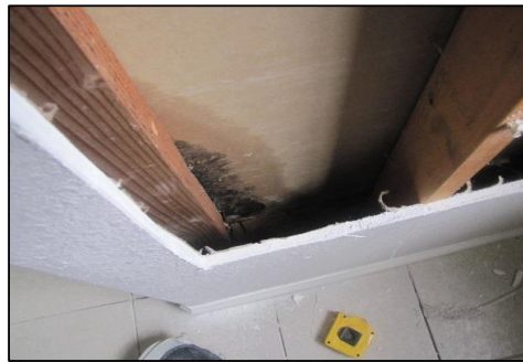
Photo # 58 Shower pan holding water and wicked off the walls past the membrane
