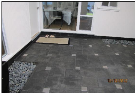
Photo # 61 Using an enhancer on a moist floor - correct: strip the old enhancer, allow the floor to thoroughly dry and reapply enhancer correctly
